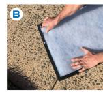
6 Install filter back into your HVAC unit following the air flow arrow; black grid facing the duct tunnel.
